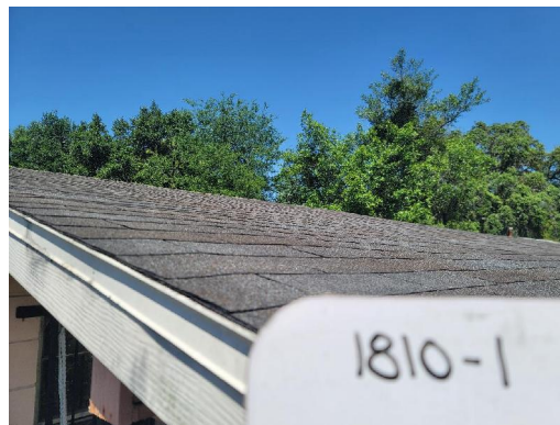
1810-1 Asphalt Shingle/Tar Typical Exterior Roof
