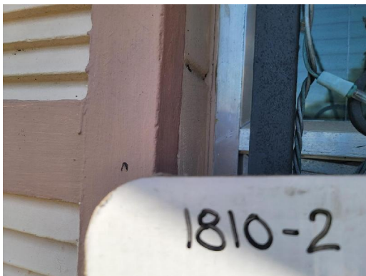
1810-2 Caulk/White (2% Chrysotile) Typical Exterior Windows
